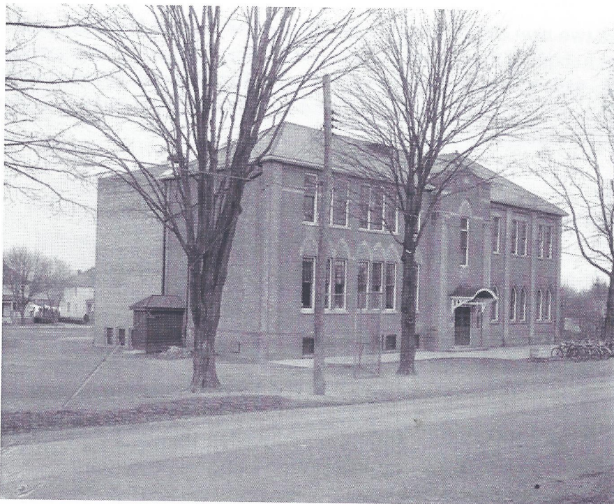
R.L. Hyslop (Saltfleet # 3) School as it appeared before closure and demolition in 1966. The original sections of the school are on the right hand side ( north ) see photos on page 3
