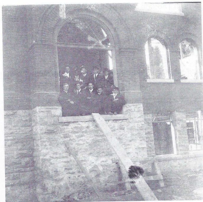
Picture during construction
