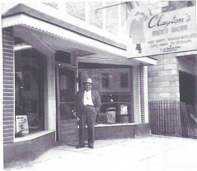
Clayton's Men's Wear built where the Blacksmith shop stood with W.S. Milmine standing out front. In the background is seen the beginning construction for the Fox theatre circa 1951.
