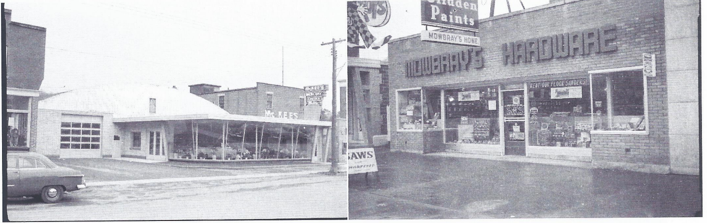
Above on the left. In the late 40's the Steel Wire factory was taken down and replaced with McKee's garage and show room and on the right Mowbray's Hardware was built in front of and attached to John Clough's Coal building shown above. It also had the building ( shown on first page ) attached to the west which was the new Royal Bank and is now Queenston Stationary.
